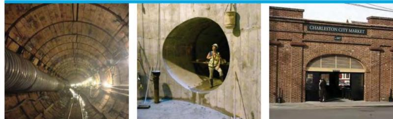
Undersized brick arches were replaced with 10-foot diameter tunnels beneath the City Market.
