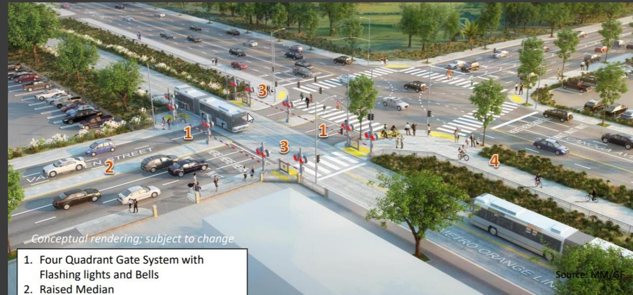
1. Four Quadrant Gate System with Flashing lights and Bells
