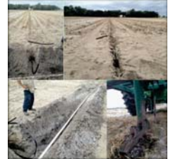
Irrigation: Installation of sub-surface drip tape
