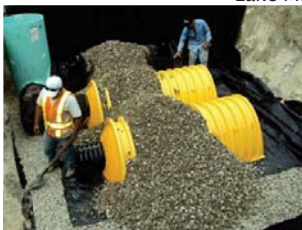
Maitland's drainage improvements
