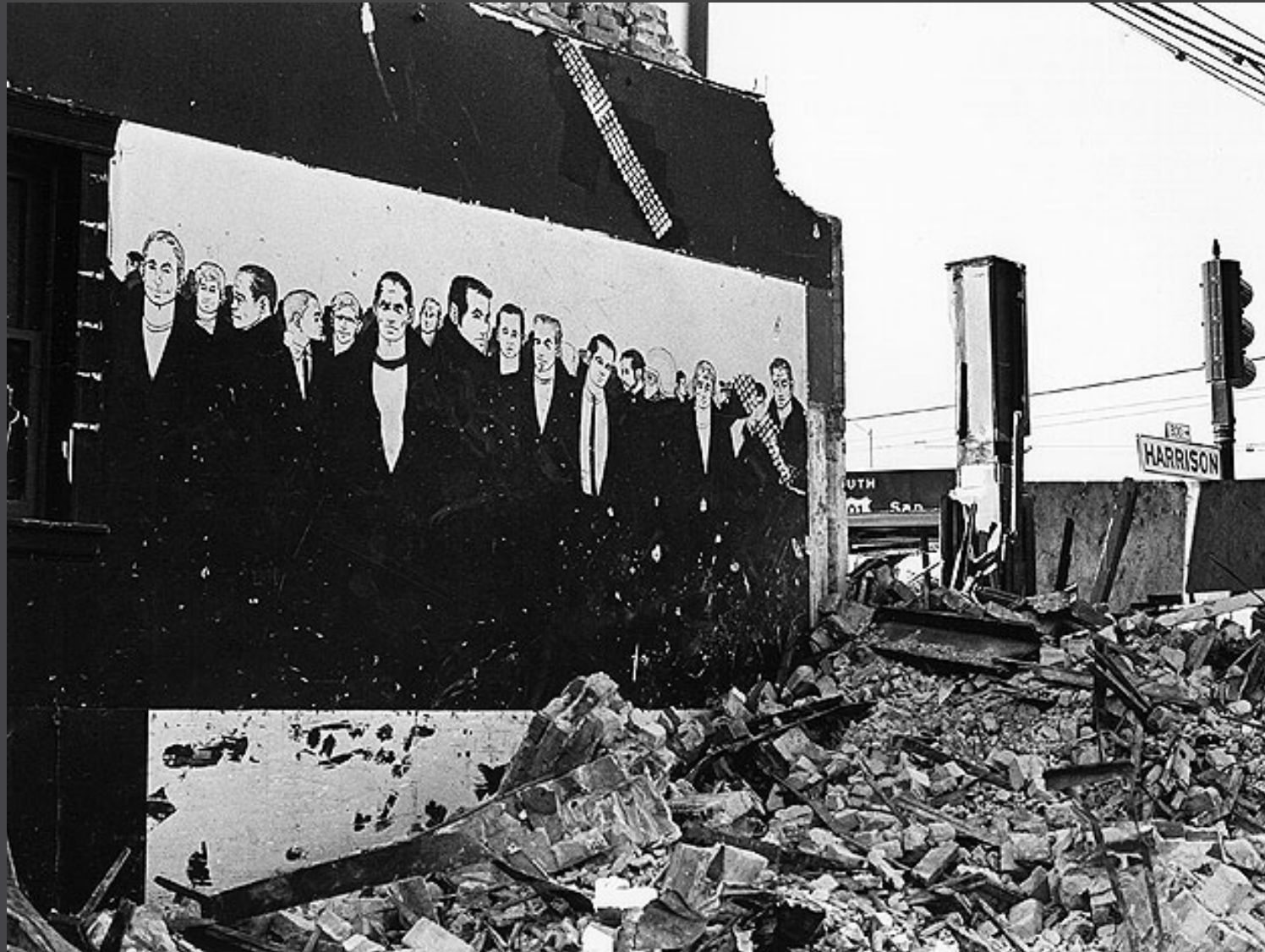
Demolition of Tool Box | 1971 (Credit: GLBT Historical Society)
