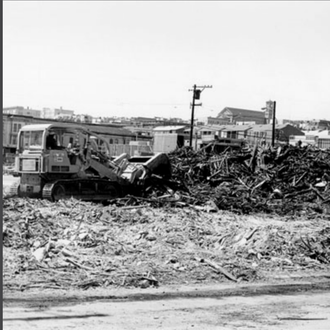
Demolition at McAllister and Laguna Streets, 1971 (Source: San Francisco Public Library)
