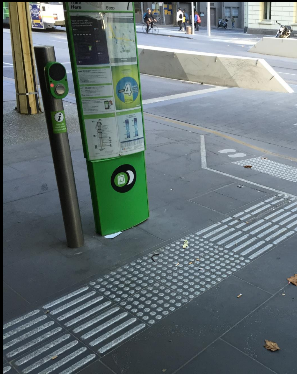
Tactile Network at Airport (specifically at transit kiosk)
