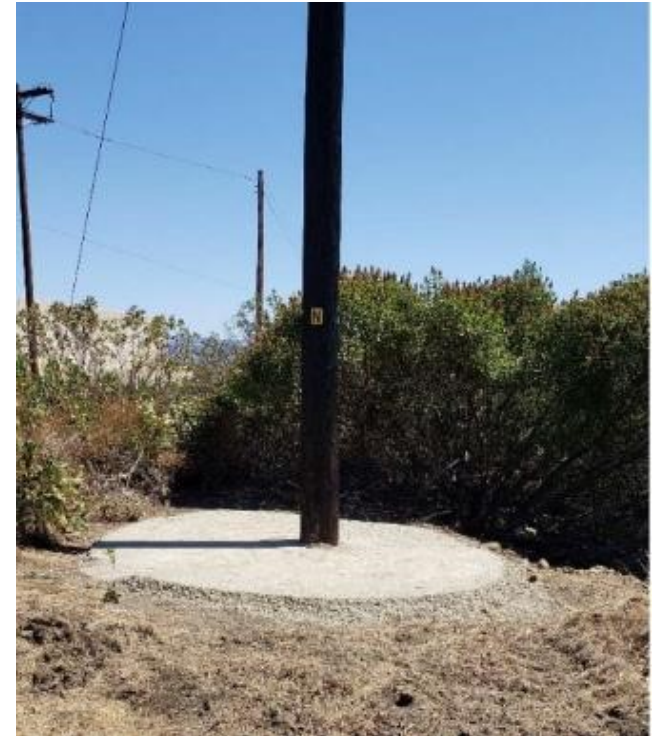
Example of 10ft clearance around distribution pole
